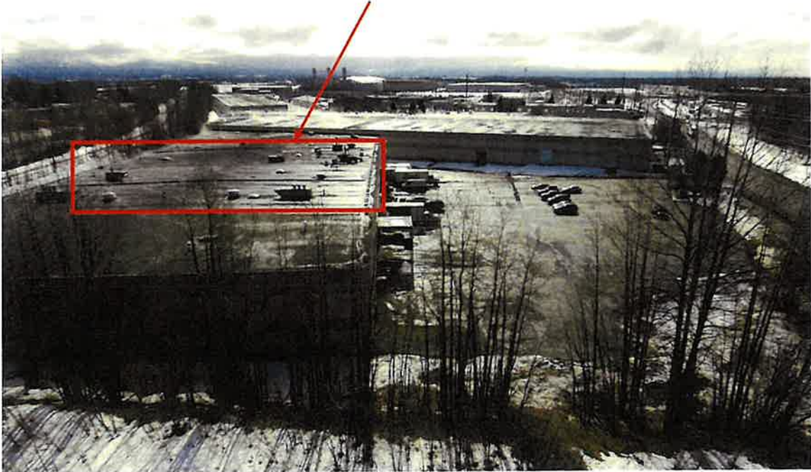
Picture 2: View from International Airport Road
