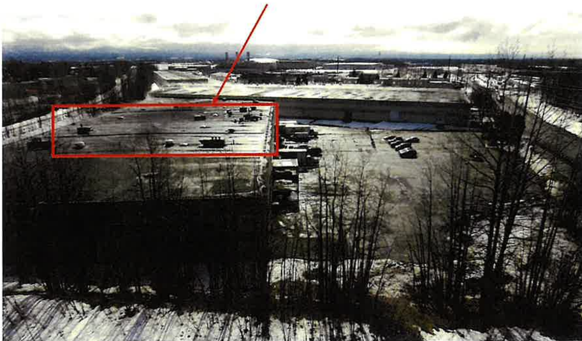
Picture 2: View from International Airport Road
